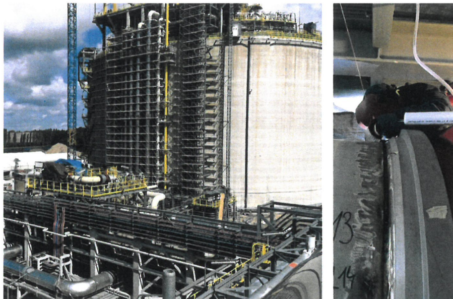
SPECIALISTIC 143 + 141 WELDINGS FOR REPAIR & GOLDEN - JOINTS - SAIPEM LNG TERMINAL - POLAND - 2015
