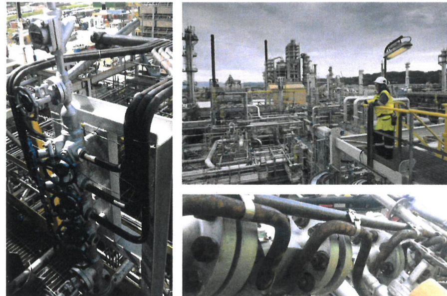
16 KM SAIPEM STEAM TRACING PIPING SYSTEM FOREMAN + PIPEFITTERS + WELDER SERVICE + TOOLS STAATSOLIE REFINERY - SURINAME 2014
