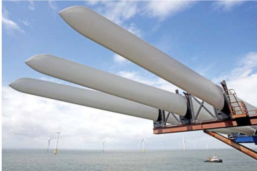
Fig. 13: Blades ready for offshore installation. Source: Siemens.
