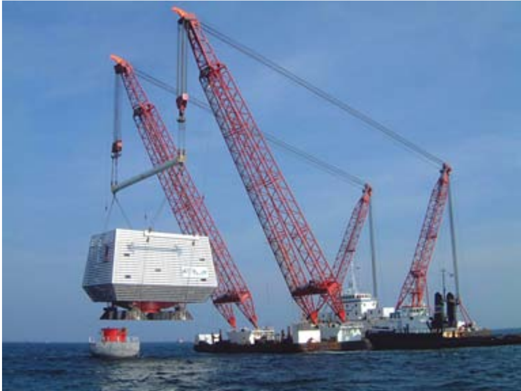
Fig. 50: Offshore transformer barge installation. Source: Repower.
