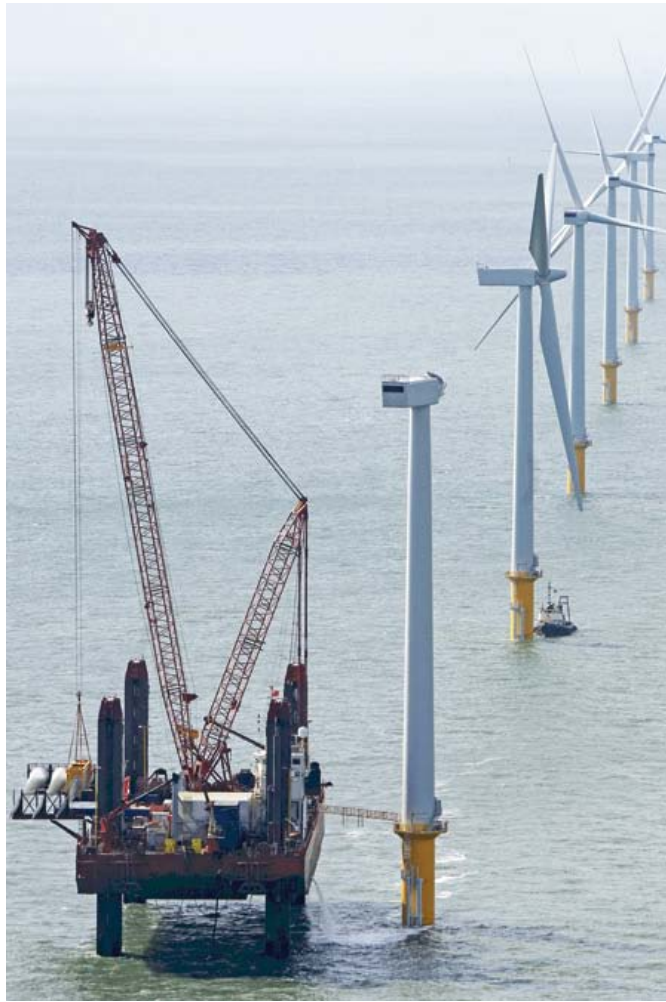
Fig. 12: Installation of the rotor blades on an offshore wind turbine. Source: Siemens.
