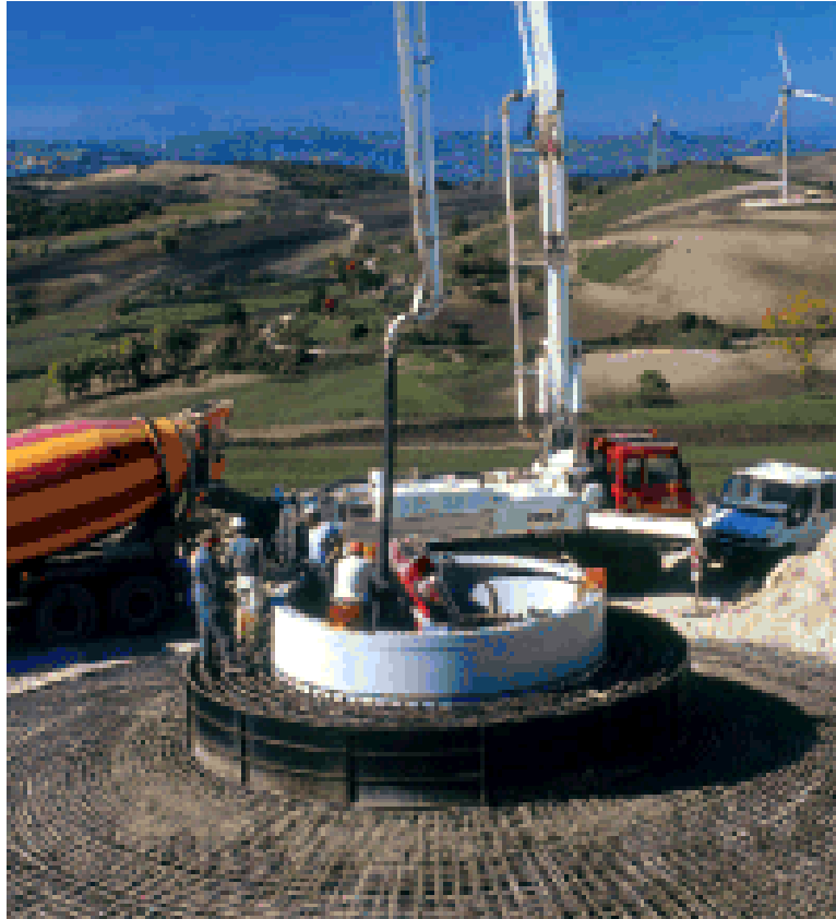
Fig. 40: Pouring of reinforced concrete into a round foundation. Source: Enercon.
