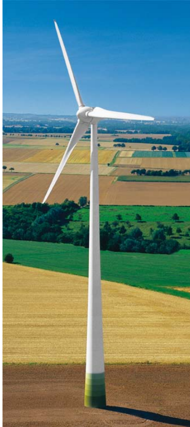
Fig. 19: Enercon E-70 2.3 MW wind turbine. The bottom of the turbine is painted in green to blend with the green surroundings. Source: Enercon.
