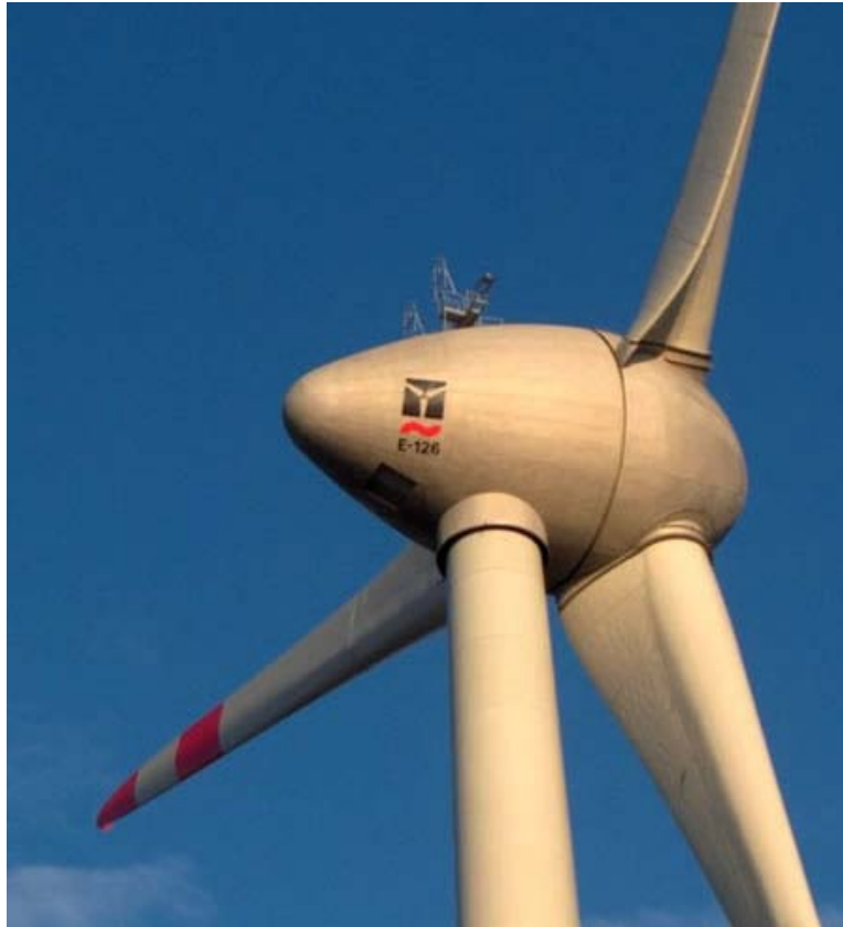
Fig. 18: Enercon E-126, 7 MW wind turbine. These turbines are equipped with a number of new features: an optimized blade design with a spoiler extending down to the hub, and a precast concrete base.
