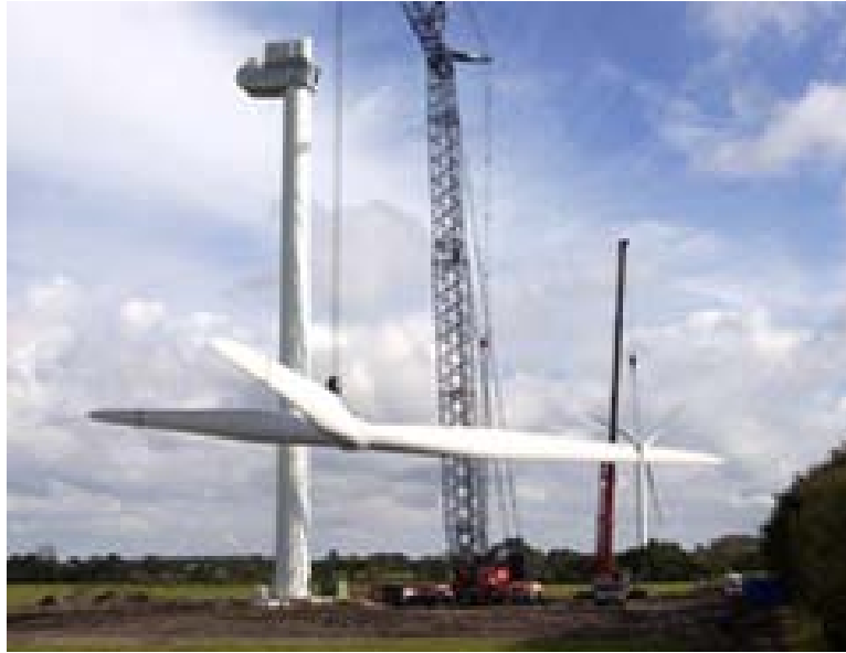
Fig. 41: Erection of a Nordex N80/2500 wind turbine. Source: Nordex.
