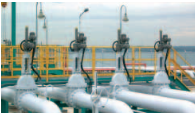
AUMA multi-turn actuators mounted on gate valves in the kerosene tank farm at Chubu airport in Japan.
