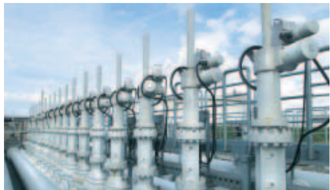
AUMA explosion-proof actuators distribute the crude oil to different tanks in a tank farm in Northern Germany.
