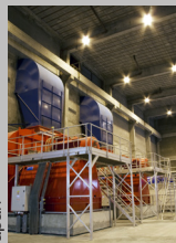
Maurice Lemaire Tunnel France
