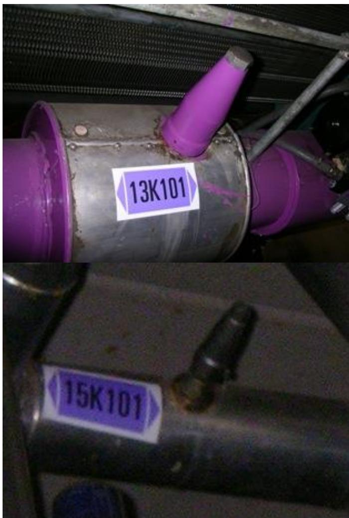
**IPOSTESI 3: FUGA AMMONIACA SEPARATORE B/P V102 SALA MACCHINE N.1****CHIUDERE VALVOLA N. 13K101 + N. 15K101 + N. 12K101**
