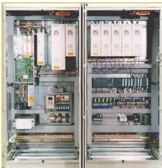
Squares command line cut sheet Fiat Cassino – Press Center (29 mt of carpentry – three PLC S7-300 319F in net – 8 panels operators – 32 drives in net – 55 encoder for positioning - about 2200 I/O)
